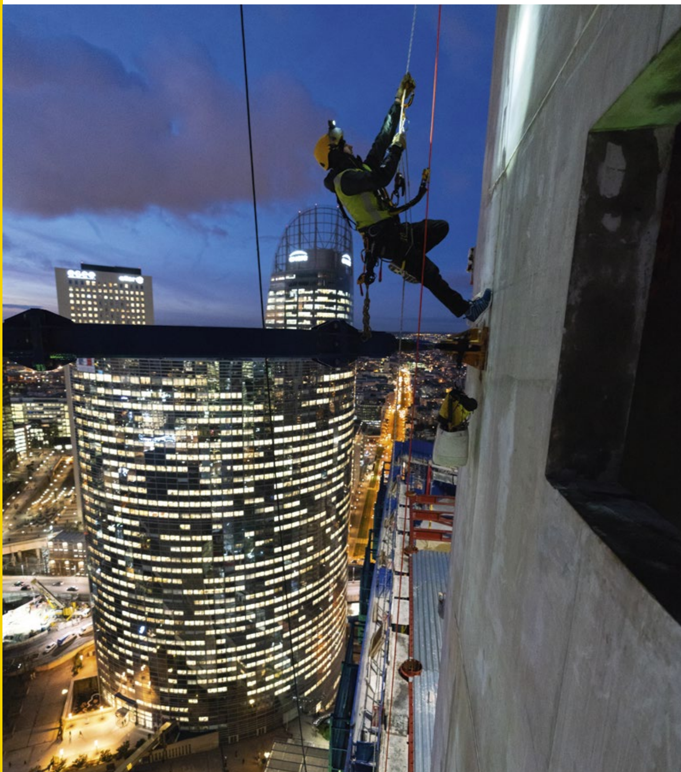
Repositioning the braces of a tower crane, France © 2019 - Petzl Distribution - Vuedici.org - Integral - Bateg - Tour Trinity - Cro&Co Architecture
